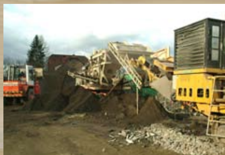
The rubble is broken down, sorted and, if possible, reused.
