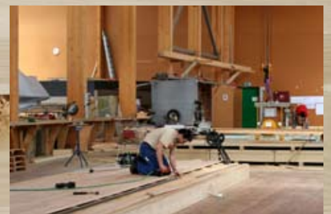
The wooden construction units are pre-fabricated by Obermayr in Schwanenstadt.
