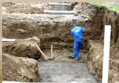
Building the foundations for the wooden support pillars.
