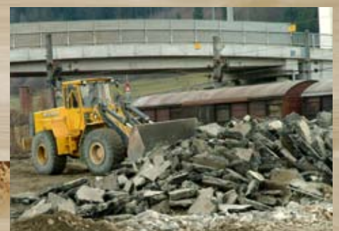
In January 2008 demolition of the old building was begun.
